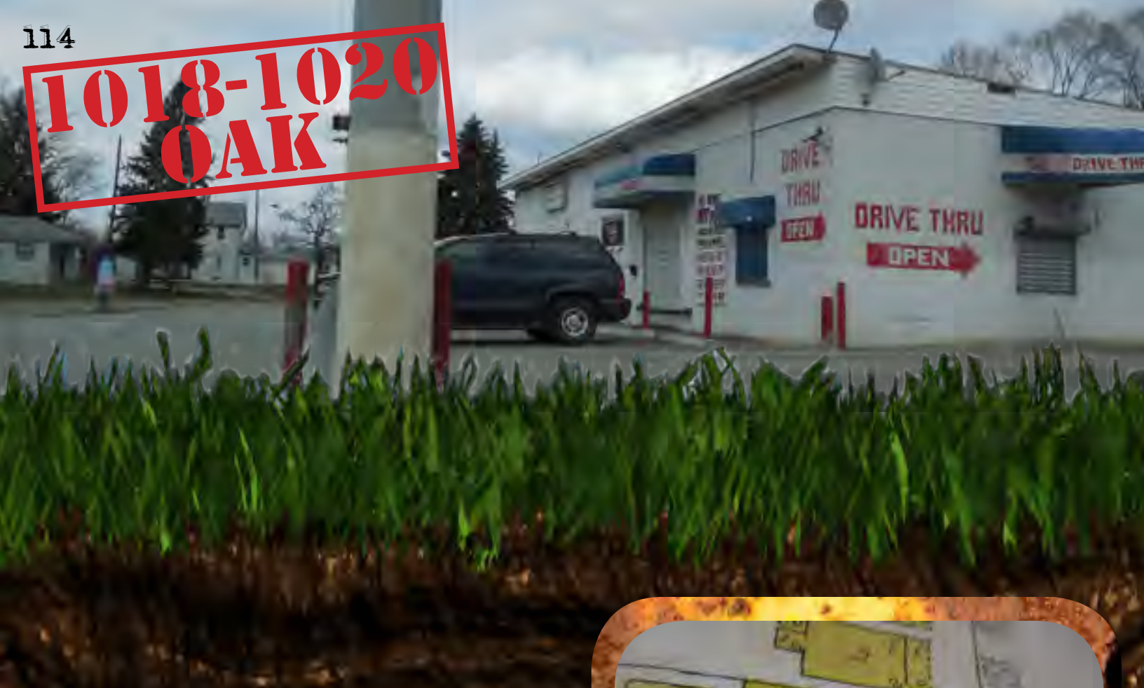
Former Gas Station
