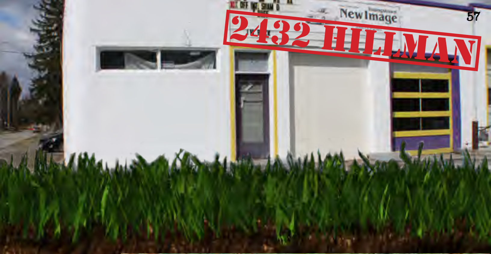
Former Gas Station
