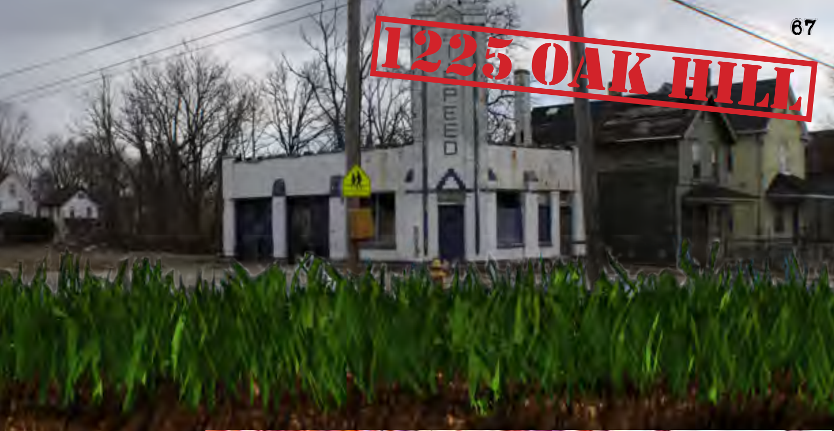
Former Gas Station
