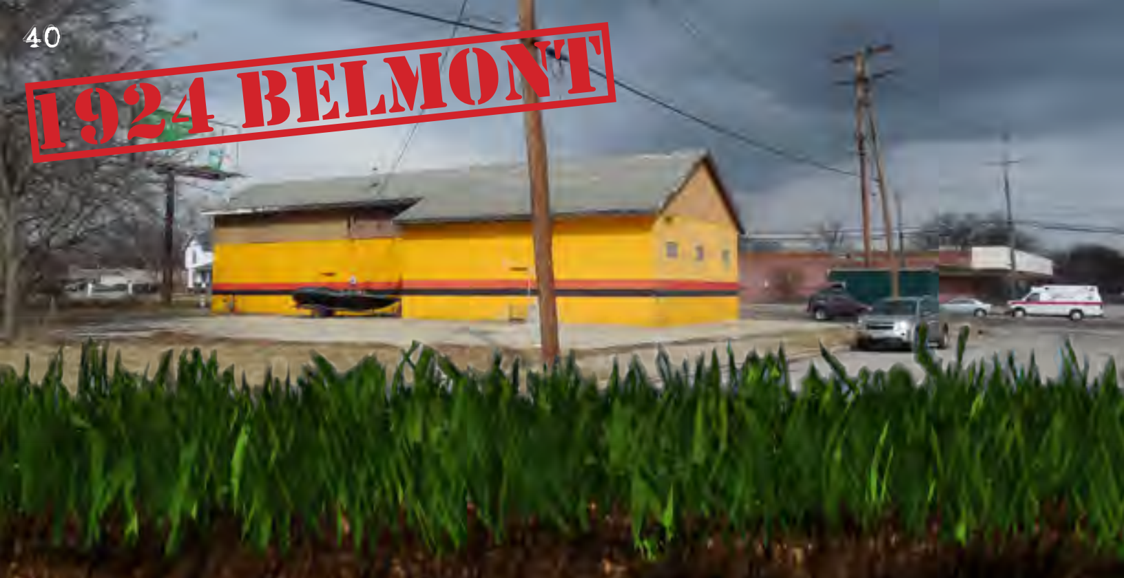
Former Gas Station
